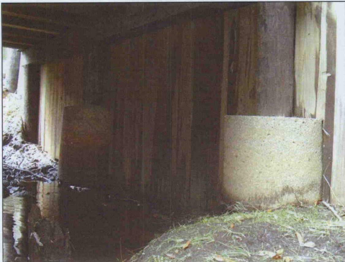
PILES 2 AND 3 AT END BENT 2 ENCASED IN CONCRETE
