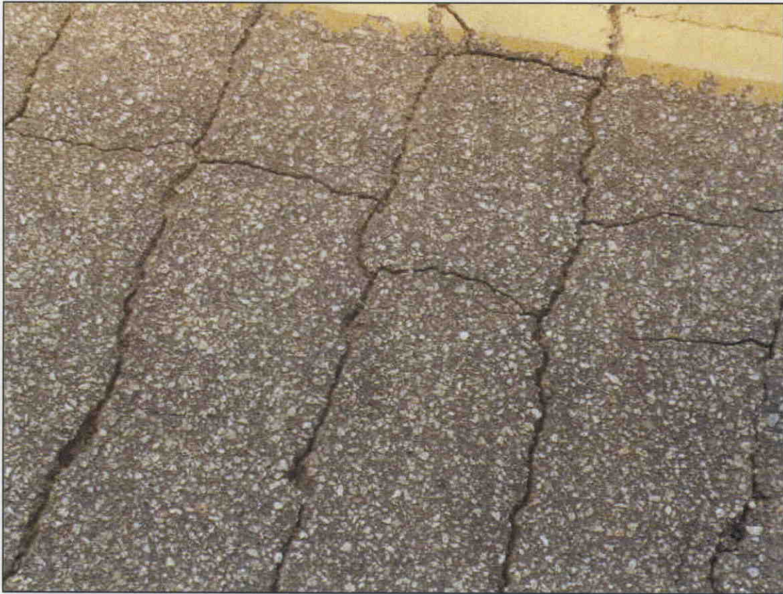
CLOSE UP OF ASPHALT WEARING SURFACE
