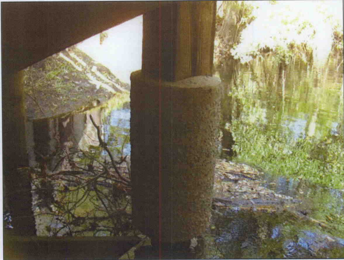
PILE 3 AT BENT 6 ENCASED IN CONCRETE
