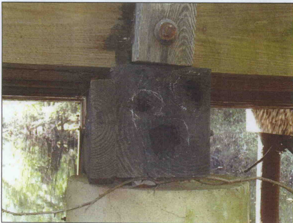
EAST END OF BENT 2 CAP DECAYED AREAS UP TO 14" LONG X 3" DIA.
