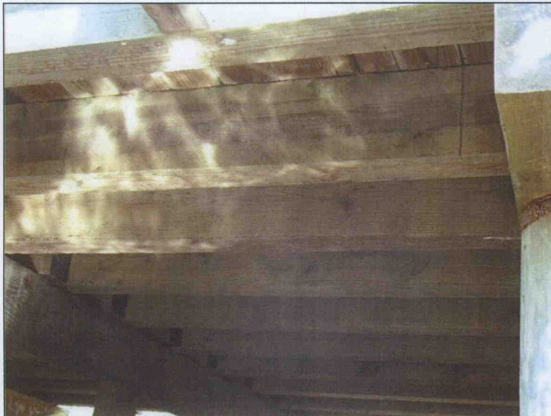
SPAN 2 UNDERSIDE ALL SPANS SIMILAR
