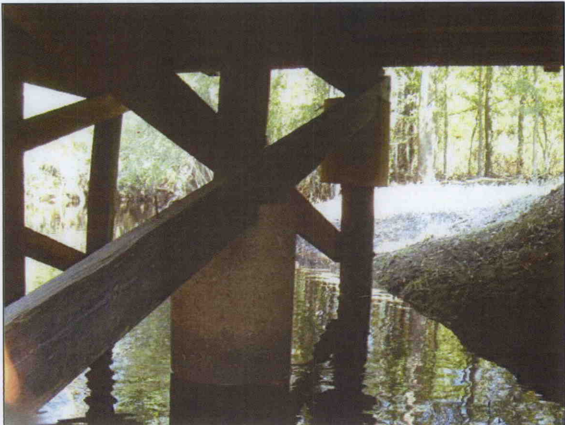
PILES 2 AND 3 AT BENT 2 ENCASED IN CONCRETE
