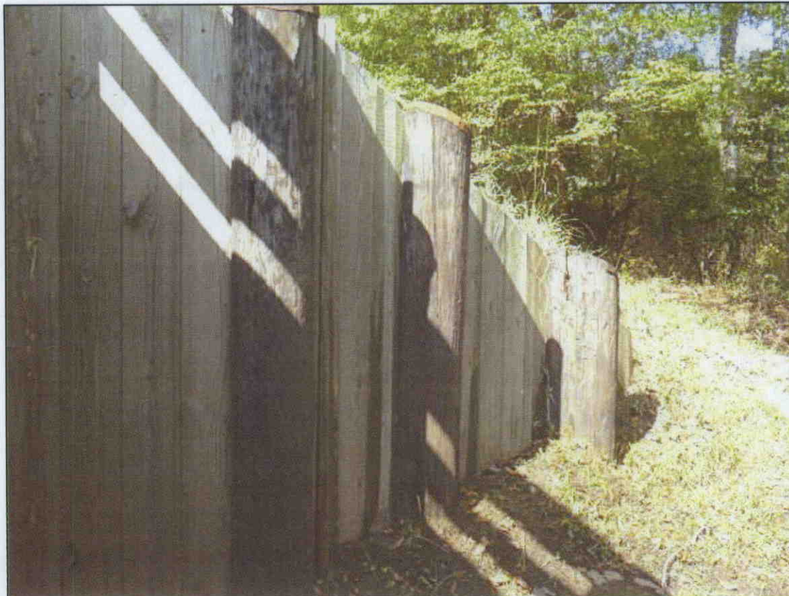
NORTHEAST TURNPILE AND WING PILE HOLLOW
