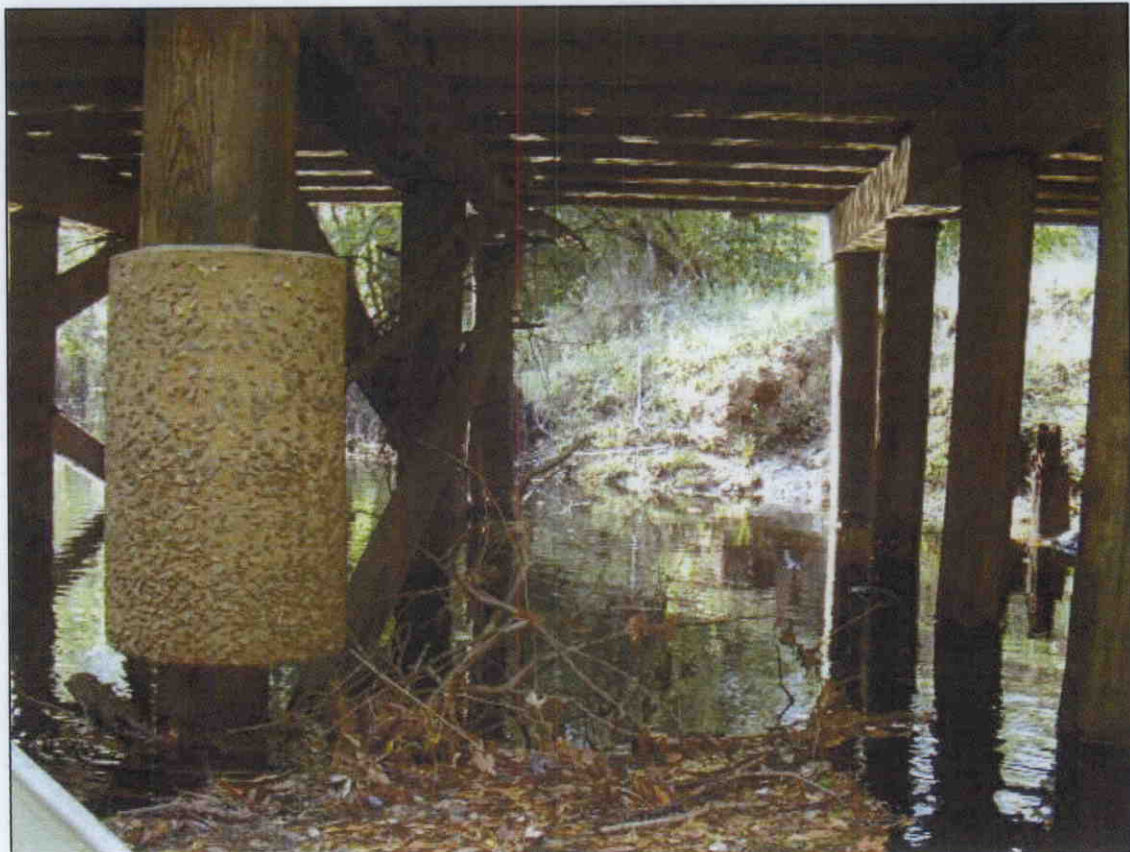
DRIFT COLLECTING AT BENT 6 UP TO 5" DIA.
