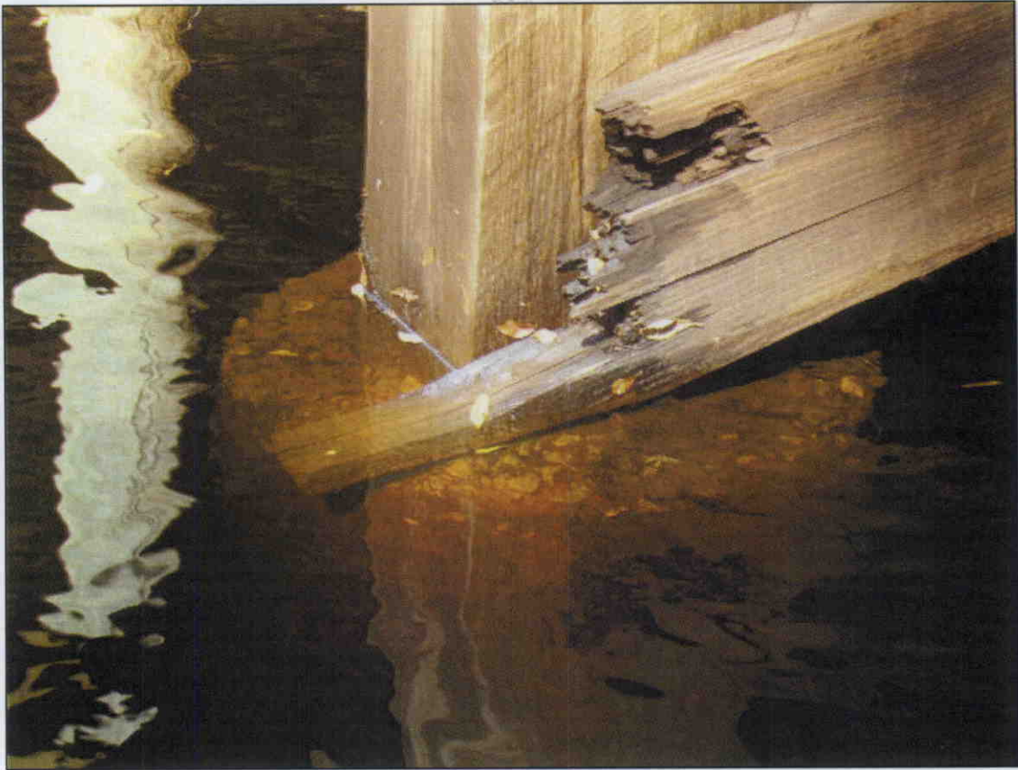
PILE 1 AT BENT 2 ENCASED IN CONCRETE
