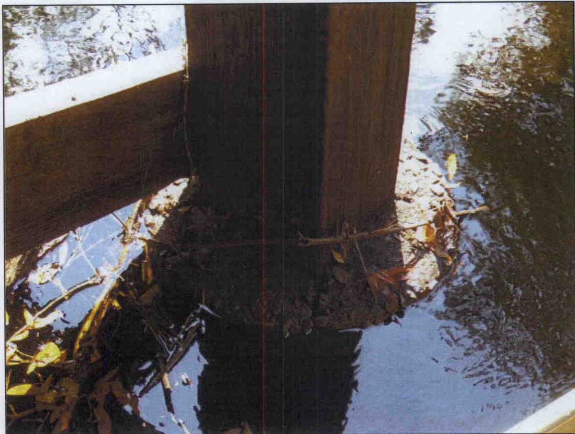
PILE 1 AT BENT 4 ENCASED IN CONCRETE
