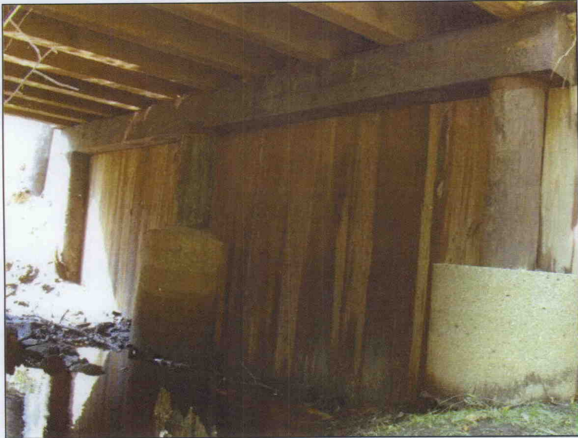
SHEET PILE BOARDS AT BULKHEAD AND WINGWALLS
